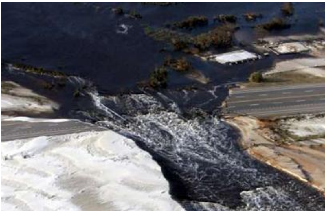
Part of a highway is washed away by receding waters in Gulf Shores, Alabama
