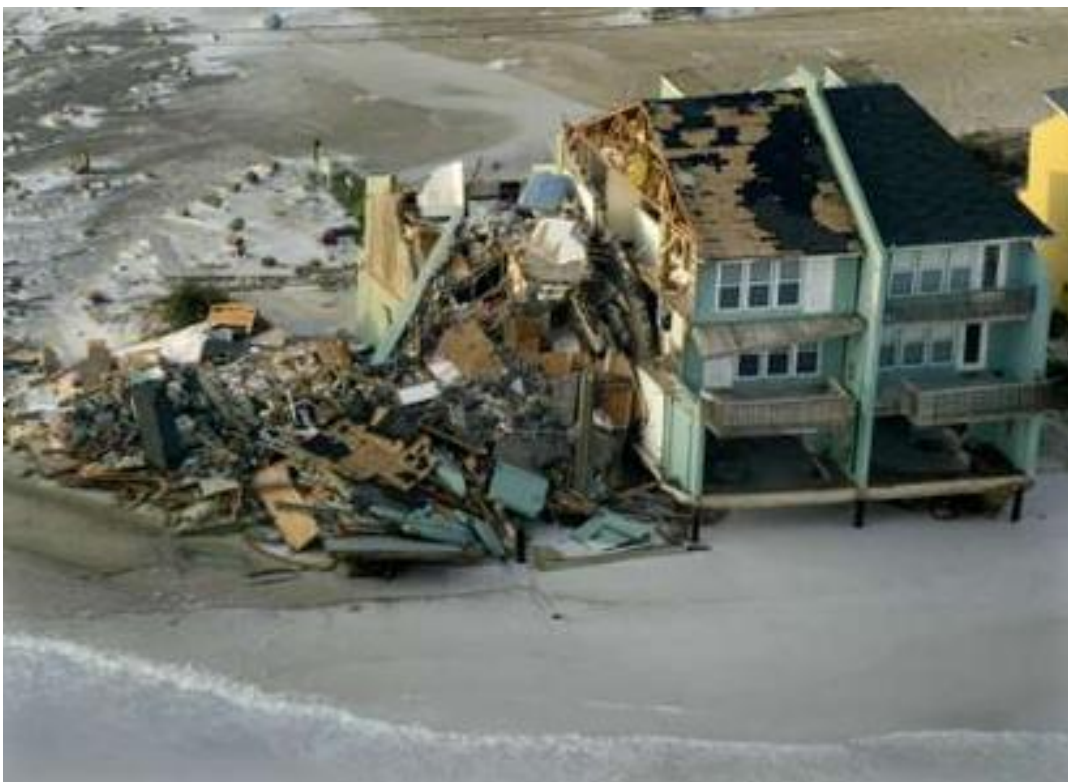
Severe damage to a building is shown in Pensacola Beach, Florida
