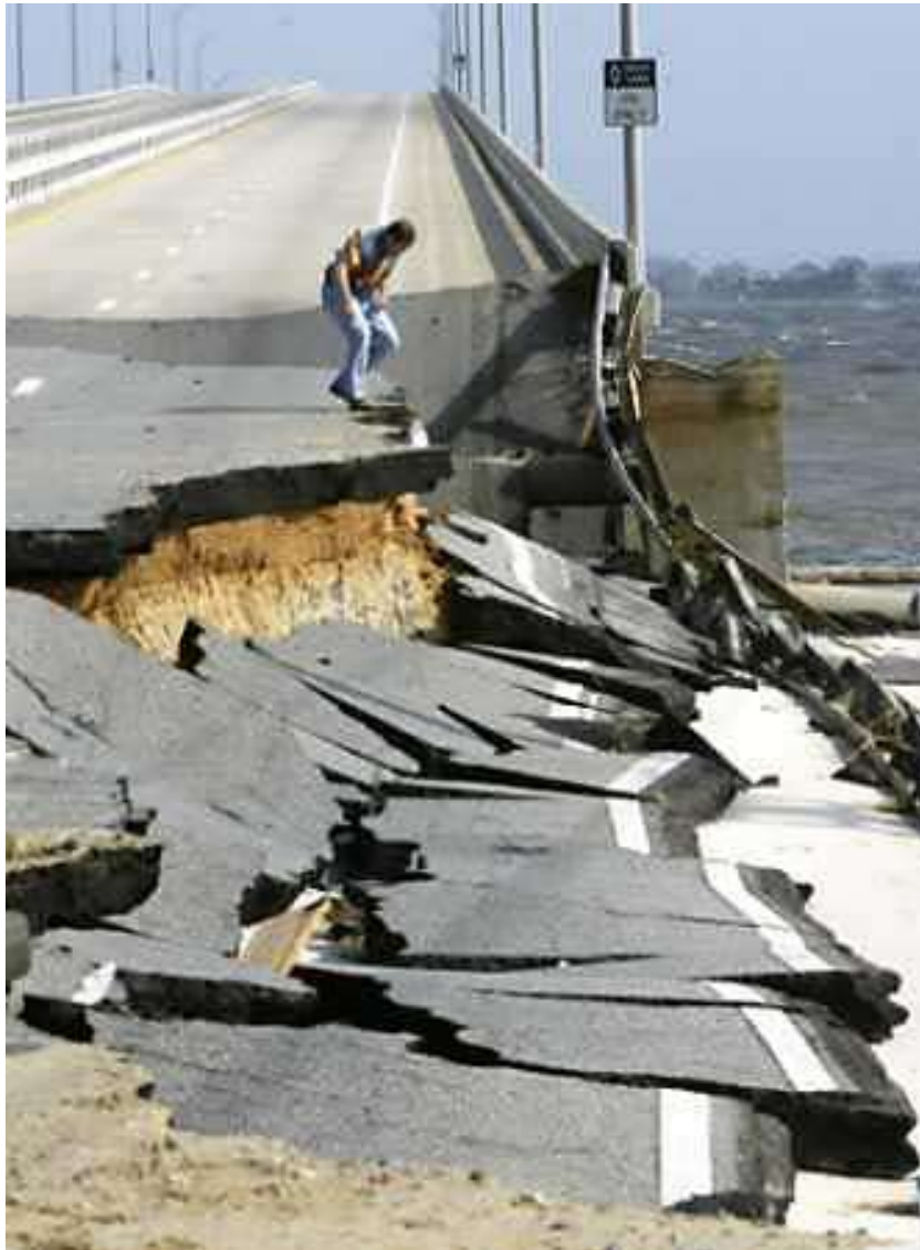
A Florida state bridge inspector looks at the destroyed bridge from Gulf Breeze, Florida to Pensacola Beach
