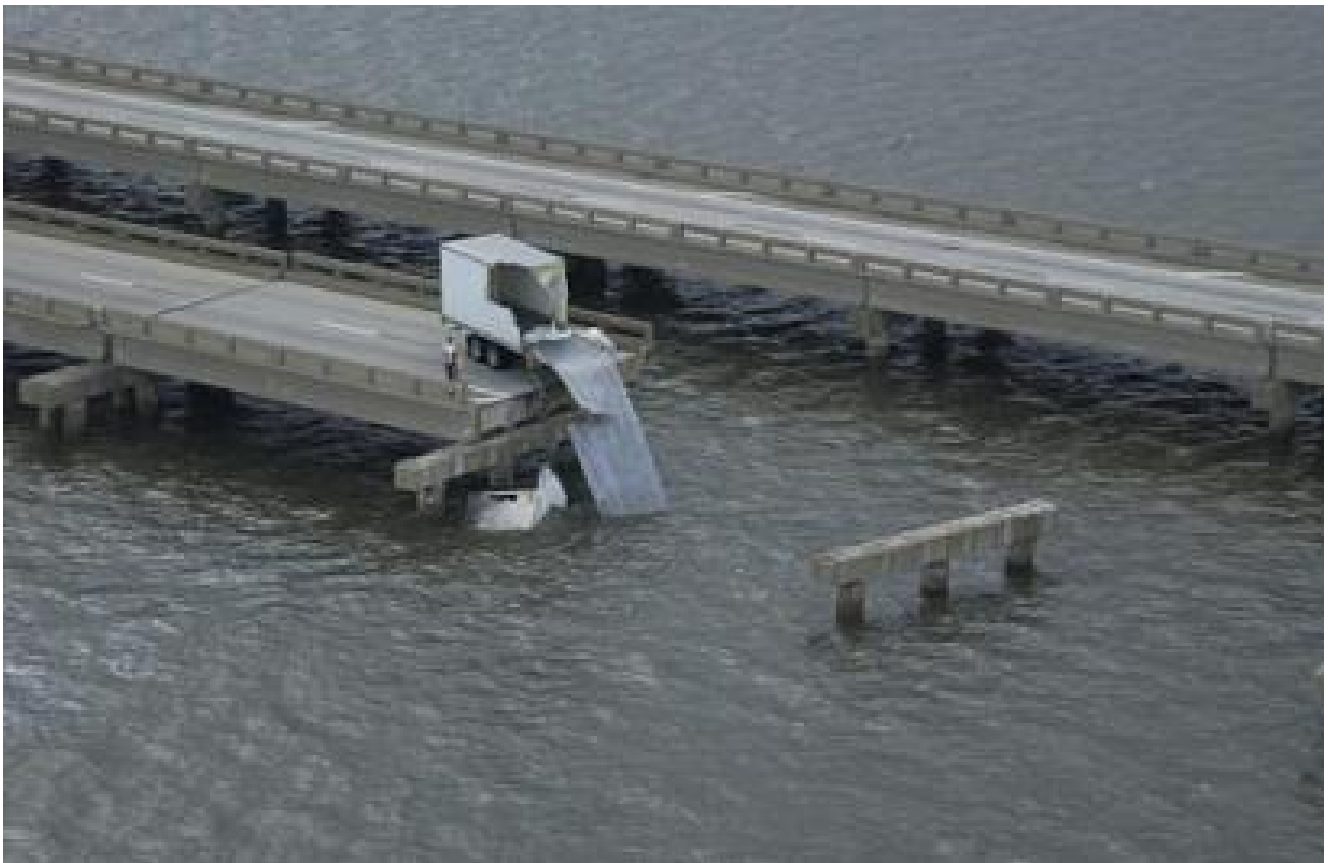
A news crew videotapes the front of a tractor-trailer that had fallen over a missing section of the Interstate 10 bridge near Pensaloca, Fla.
