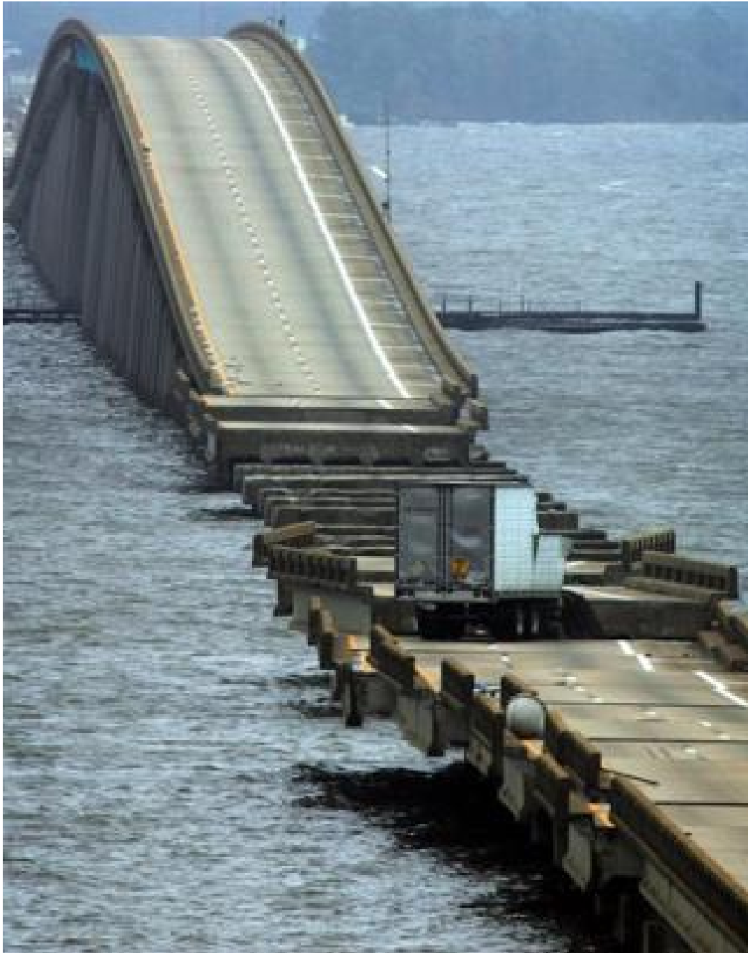
A tractor trailer rests on a section of I-10 bridge that crosses Escambia Bay, in Pensacola, Fla
