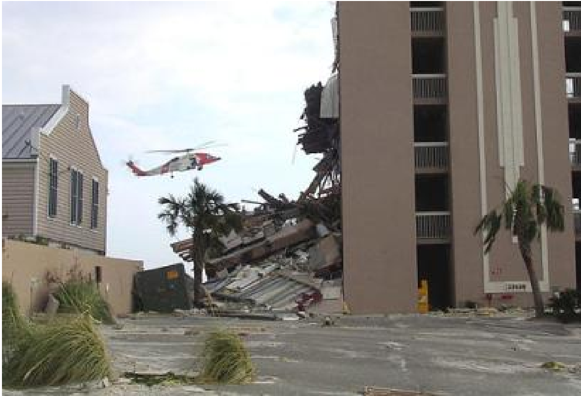
A U.S. Coast Guard helicopter flies past the remains of a condominium tower that partially collapsed in Orange Beach, Ala
